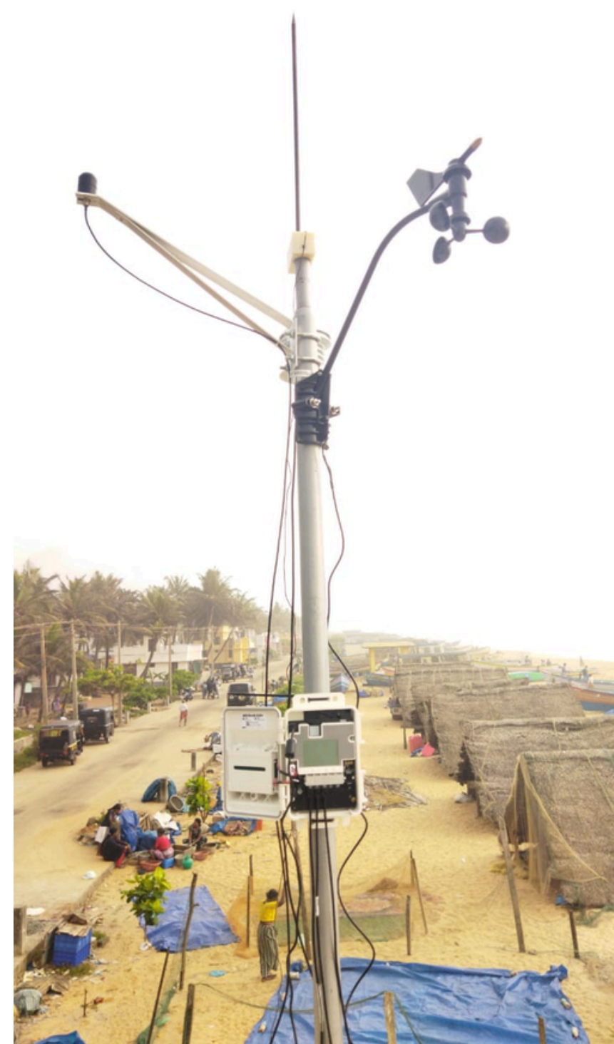
Fig. 14.5.14. Early warning system installed near coast for weather pattern shifts
