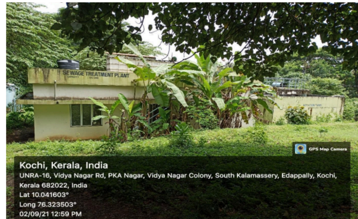
Fig. 14.5.25. Sewage treatment plant at CUSAT
