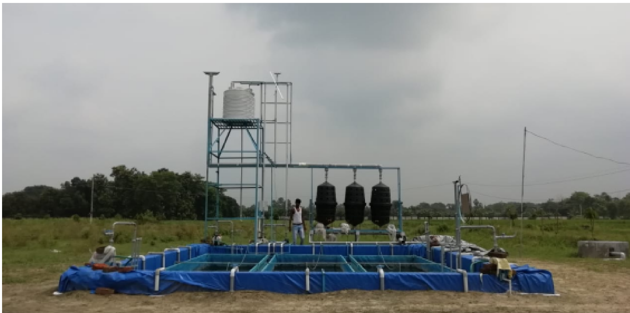
Fig. 14.5.18. Recirculating Aquaculture Systems (RAS) installed by NCAAH, CUSAT
