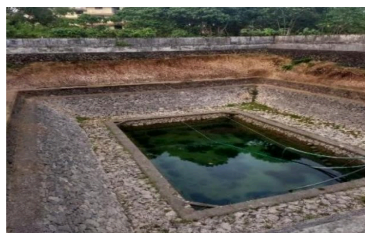
Fig. 14.5.23. Constructed Tanks and Bunds for water conservation at CUSAT
