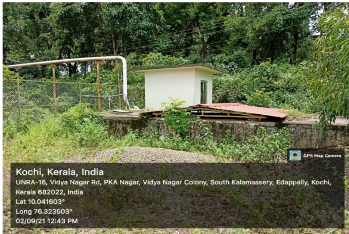
Fig. 14.5.20. Water treatment plant at CUSAT
