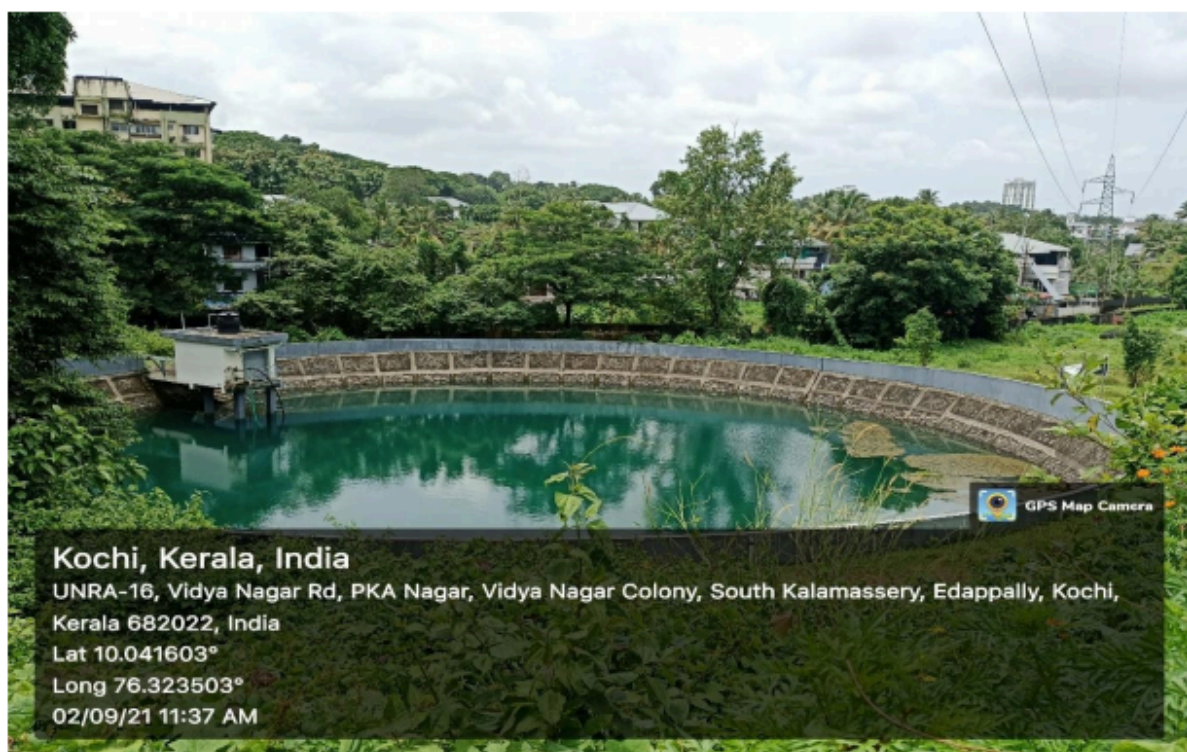
Fig. 14.5.24. Rainwater Harvesting at CUSAT
